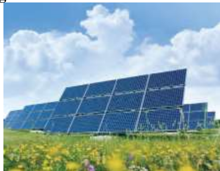
Figure 13: Photovoltaic Solar Energy
